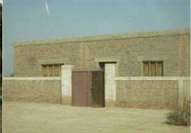
Figure 5.6: View of SIDA Building
